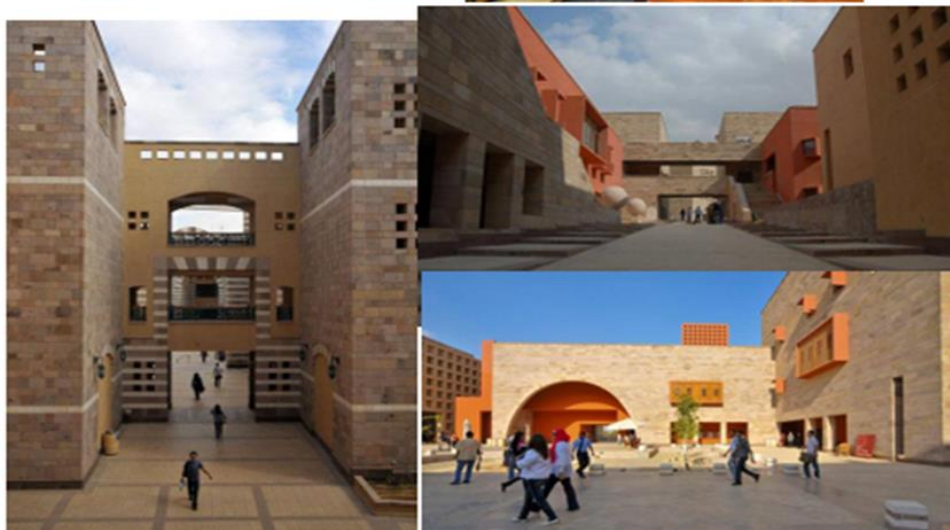
pic Nos. (29, 30, 31, 32, 33 and 34) indicating the internal and external design of the American University in Cairo, Reported by http://archnet.org/sites/6717/media_ contents/ ArchNet
