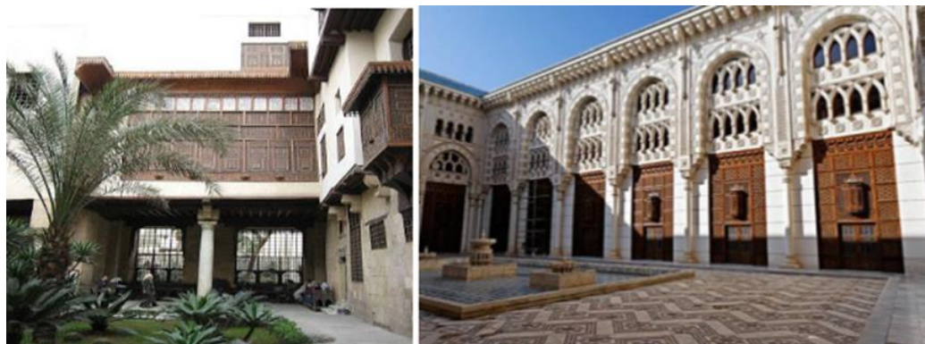
pic Nos. (14 and 15) indicate the variety of building methods in Islamic architecture. Reported by http://wagihyoussef.tumblr.com/
